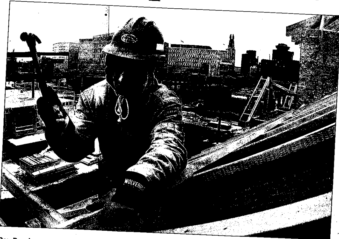
Ron Rossborough of Mark IV Construction nails in a roof-rafter brace on Tuesday at the Corn Hill Landing complex. Even though the facility won't open until June, tenants are already lining up. JAY CAPERS staff photographer
